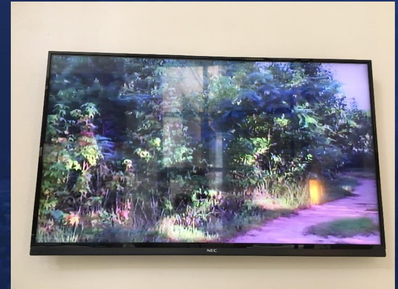
Installed 11 video monitors around the facility
