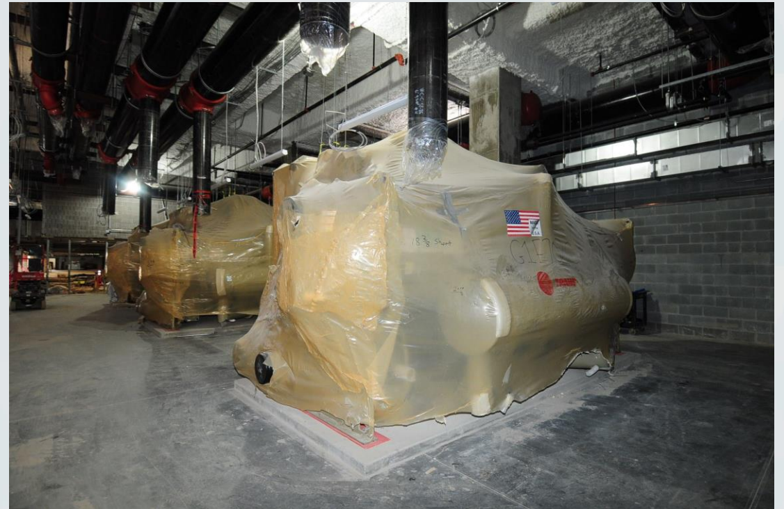
CEP – Chiller Progress
