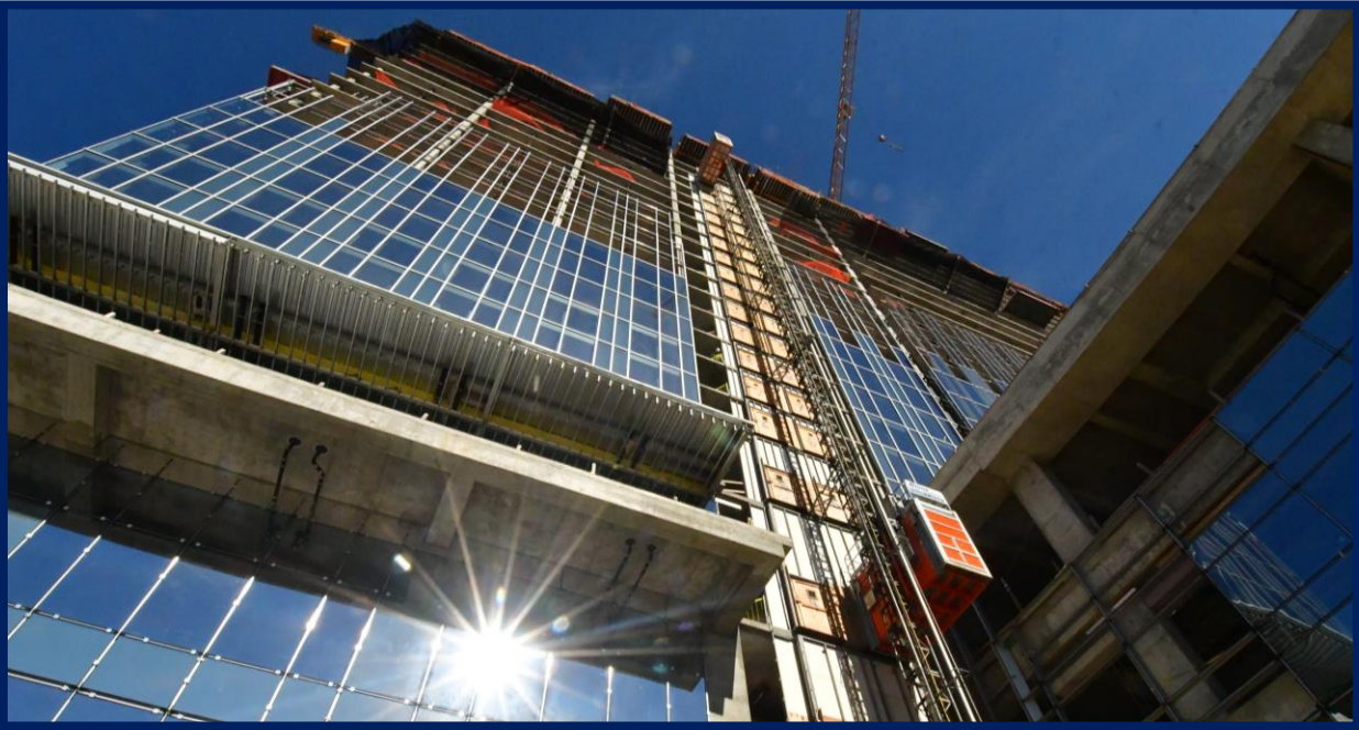
Curtainwall Installation
